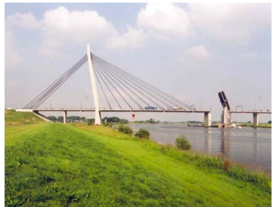
Eilandbrug at Kampen/Netherlands with dampers of type SDE-V
