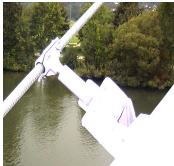
SDE-R installed in the bridge Forchheim
