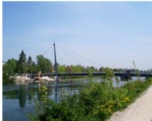
Traunsteig in Wels/Austria with cable dampers of type SDI-R
