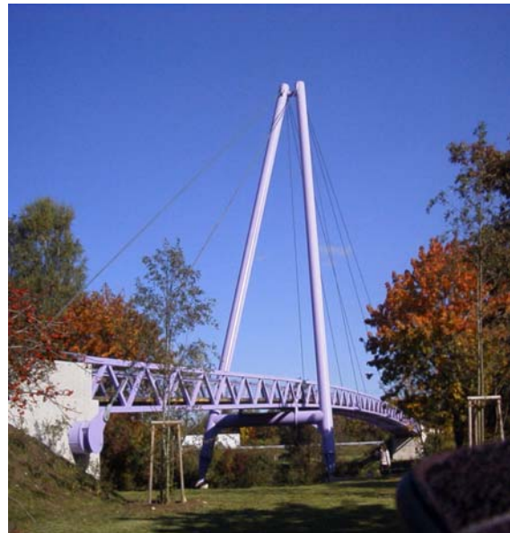
Footbridge Forchheim/Germany with SDE-R cable dampers at the stay cables
